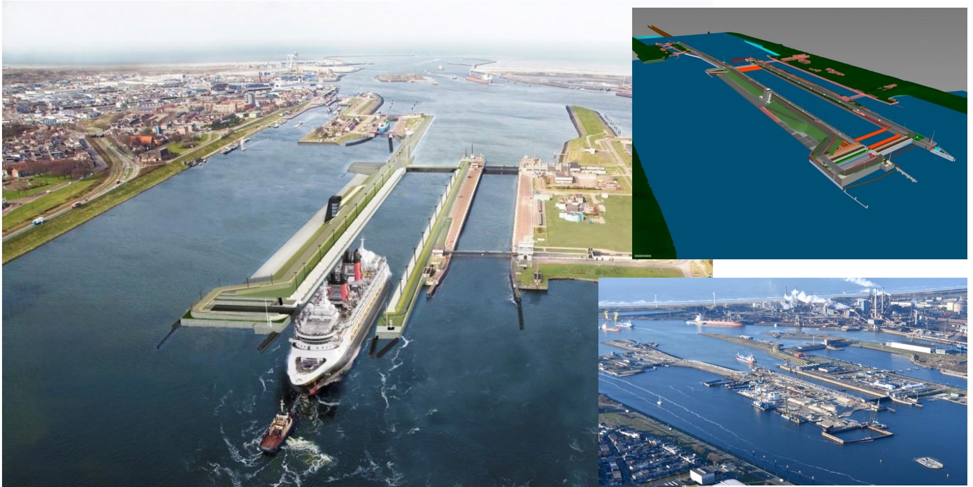
Sea lock North Sea Canal – IJmuiden – The Netherlands
